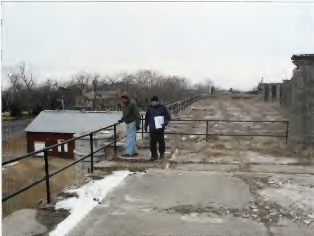
Figure 3.30. View looking north across terreplein, Battery Potter. As an additional safety measure, guardrails are installed on the western portion of the terreplein to prevent access to the sloped portion of the concrete structure (Olmsted Center, January 2009).
